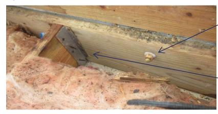
Wood roof member bolted to masonry wall and clip with at least 3 nails into the rafter
