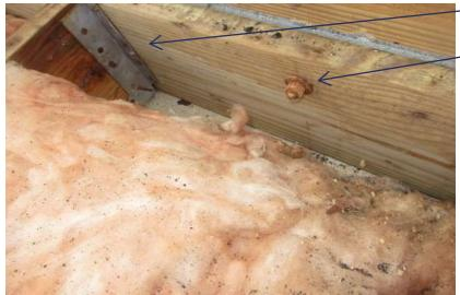
Wooden roof member bolted to masonry wall and clip with at least 3 nails into the rafter
