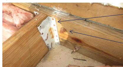
Wooden roof member bolted to masonry wall and clip wtih at least 3 nails into the rafter
