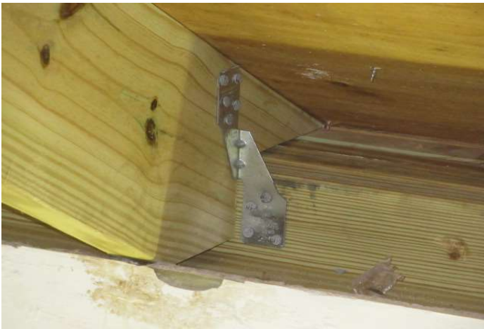
Clips with at least 3 nails into the rafter
