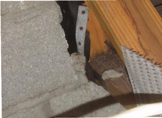
Flat roof truss resting in the masonry exterior wall, held in place with strap with at least 3 nails
