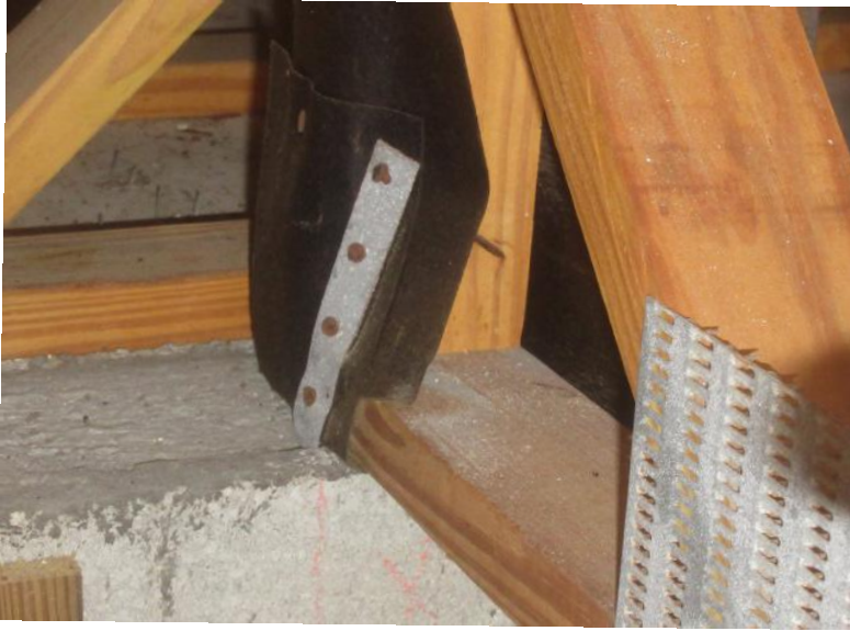
Flat roof truss resting on exterior masonry wall and attached with strap with at least 3 nails
