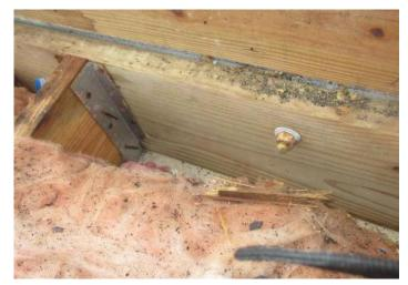
Ledger board bolted to exterior masonry wall and rafter attached with clip with at least 3 nails
