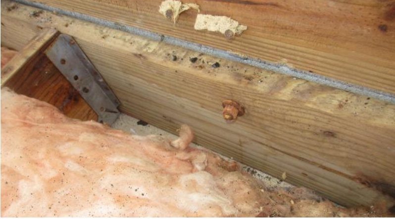
Ledger board bolted to exterior masonry wall and rafter attached with clip with at least 3 nails
